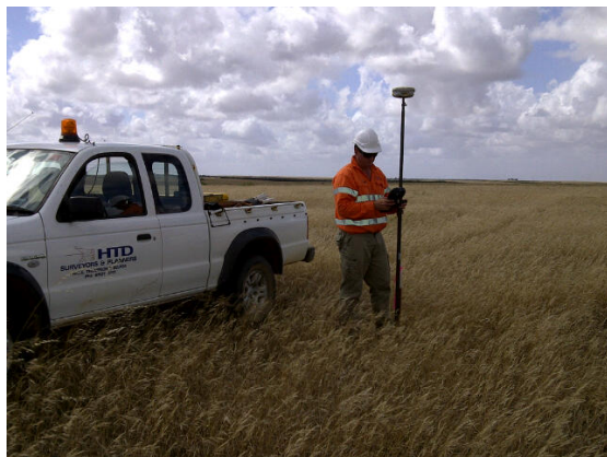
Surveying the site.
