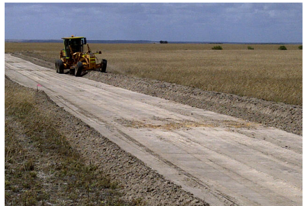
Grading roads at the solar farm site.
